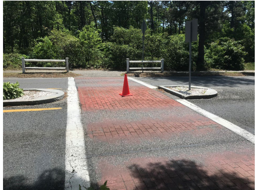
Figure 205: Raised and Stamped Brick Crosswalk Improves Visibility. Bricks are Faded However.
