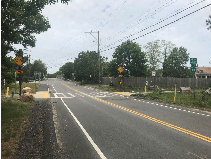
Figure 200: Ladder Crosswalk, Bike Trail Crossing Signs, Advance Bike Trail Crossing Signs, RRFBs, and Clear Sightlines Make Crossing Highly Visible
