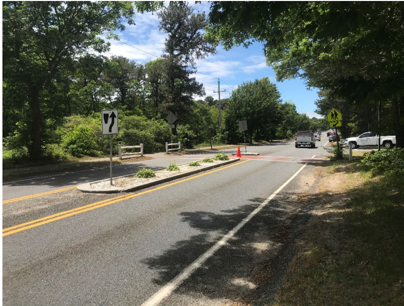
Figure 204: Westbound View of the Crosswalk with Median to Allow 2-Stage Crossings
