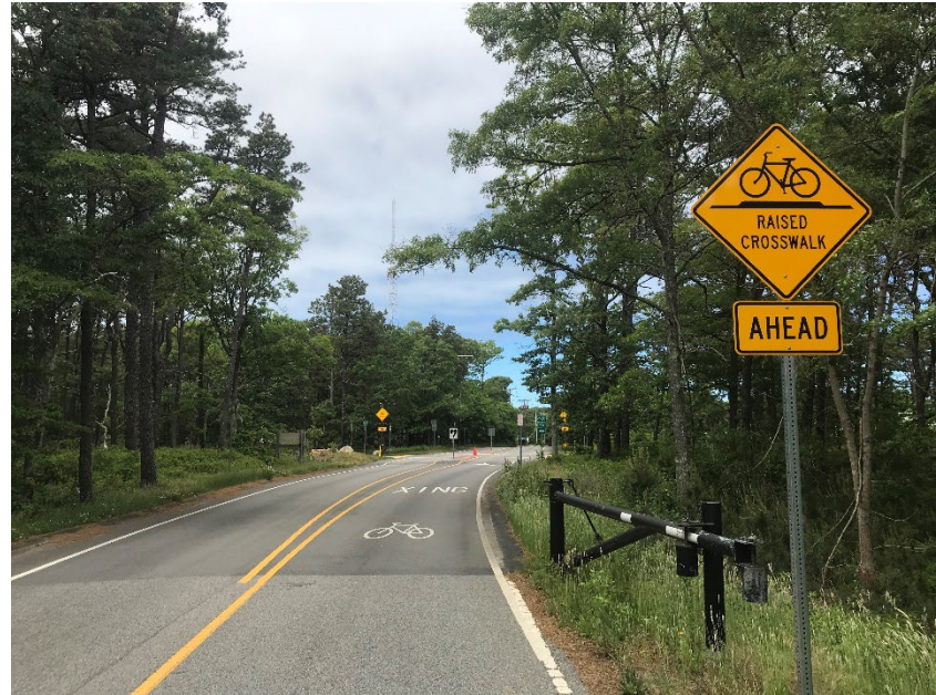
Figure 203: Raised Crosswalk Ahead Signage, Along with Sharrows Demonstrating Bicyclist Crossings
