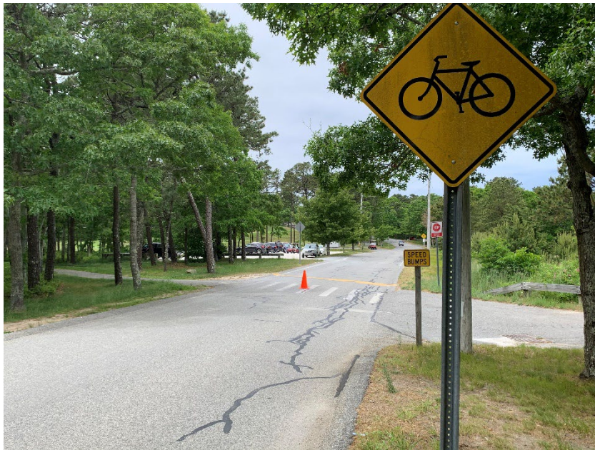
Figure 210: Westbound Road Approach with Speed Bumps, Faded Crosswalk, and Faded Shared Use Path Signage
