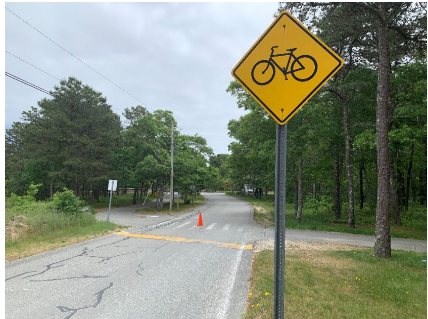
Figure 211: Eastbound Road Approach with Speed Bumps, Faded Crosswalk, and High-Quality Shared Use Path Signage
