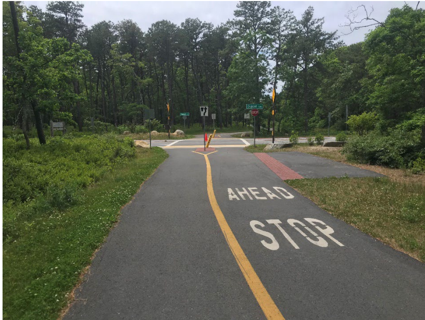
Figure 202: High-Quality Advance Pavement Markings, with a Splitter and Clear Lines of Sight
