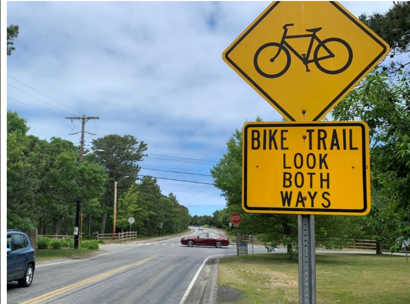
Figure 209: Image Looking Northward; Advance Bike Trail Crossing Signage Improves Awareness of Crossing on Both Approaches
